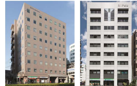
Win Gotanda Building 2 (Shinagawa-ku, Tokyo)
