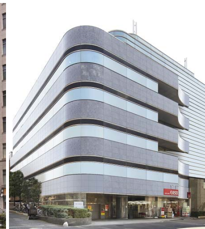
Ichigo Hongo Building
