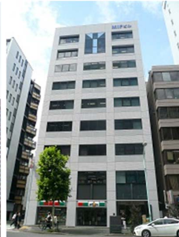
MIF Building (Tokyo)
