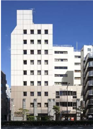
Ichigo Mita Building (Minato-ku, Tokyo)
