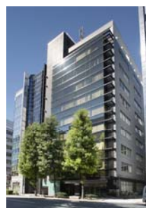
Ningyocho Central Building
