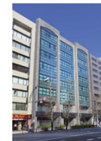
Ichigo Akihabara North Building
