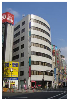
Kichijoji Central Building (Tokyo)
