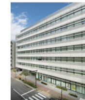
Ichigo Nihonbashi East Building
