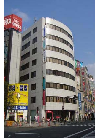
Kichijoji Central Building (Tokyo)
