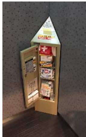
Elevator Emergency Supply Cabinet
