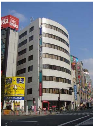
Kichijoji Central Building (Tokyo)
