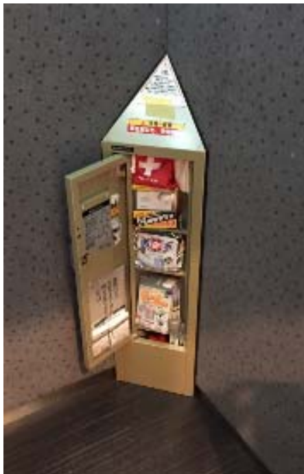
Elevator Emergency Supply Cabinet
